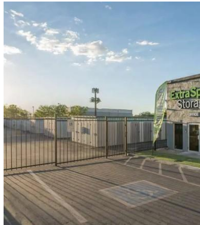
Tempe, Arizona, self-storage
